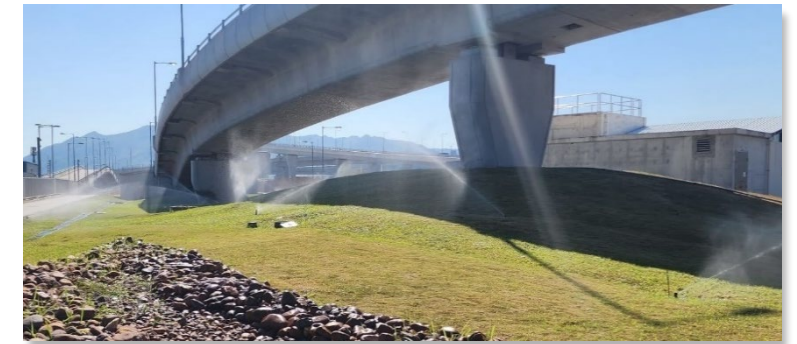
Irrigation by rainwater harvest system at HZMB HKP
